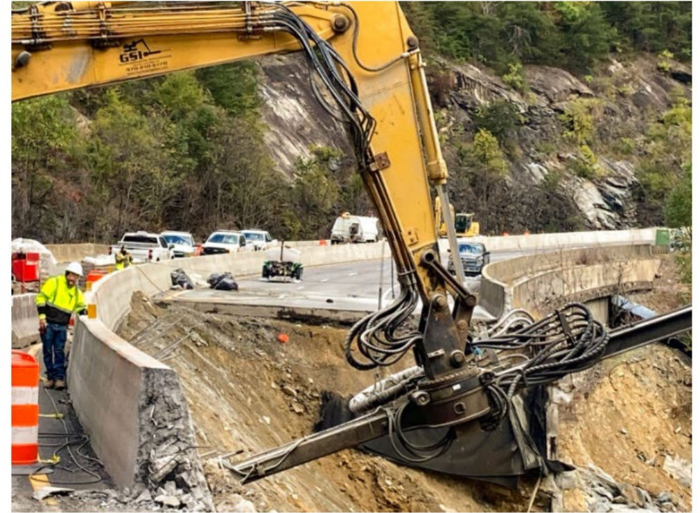
NCDOT crews worked to shore up the Pigeon River gorge last October — one of the first steps toward rebuilding Interstate 40 near the Tennessee border. (Photo by NCDOT)
