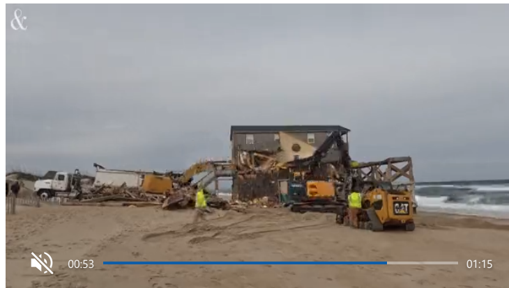
Crews demolish beach homes on NC Outer Banks
