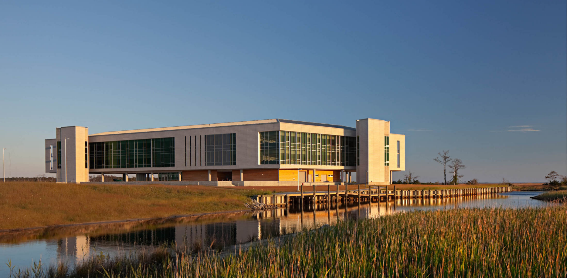
view from northwest along new canal
